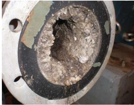
Figure 2 - Example of struvite deposition in a pipe from anaerobic digester (Bergmans 2011)
